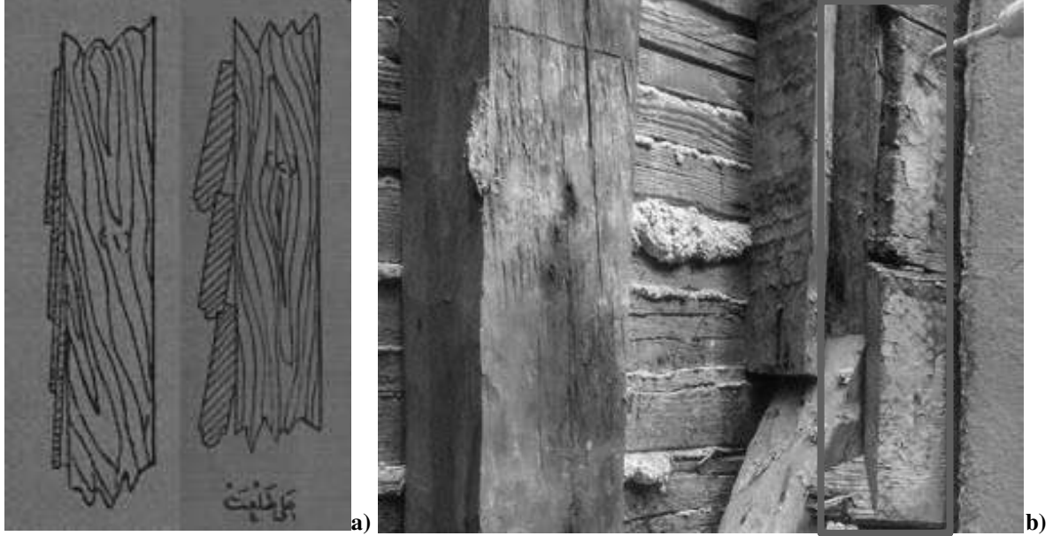
Figure 3. Timber façade covering boards from a) Ali Talat drawings [3] and b) Tuzcuğlu House at Beylerbeyi [4]
