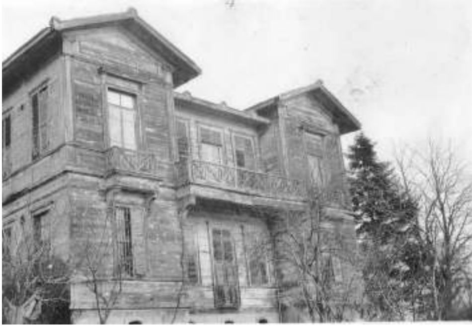
Figure 5: Prefabricated timber house constructed for Prince Vahdettin in Çengelköy (Istanbul Protection Board, Encümen Archive, 1955)
