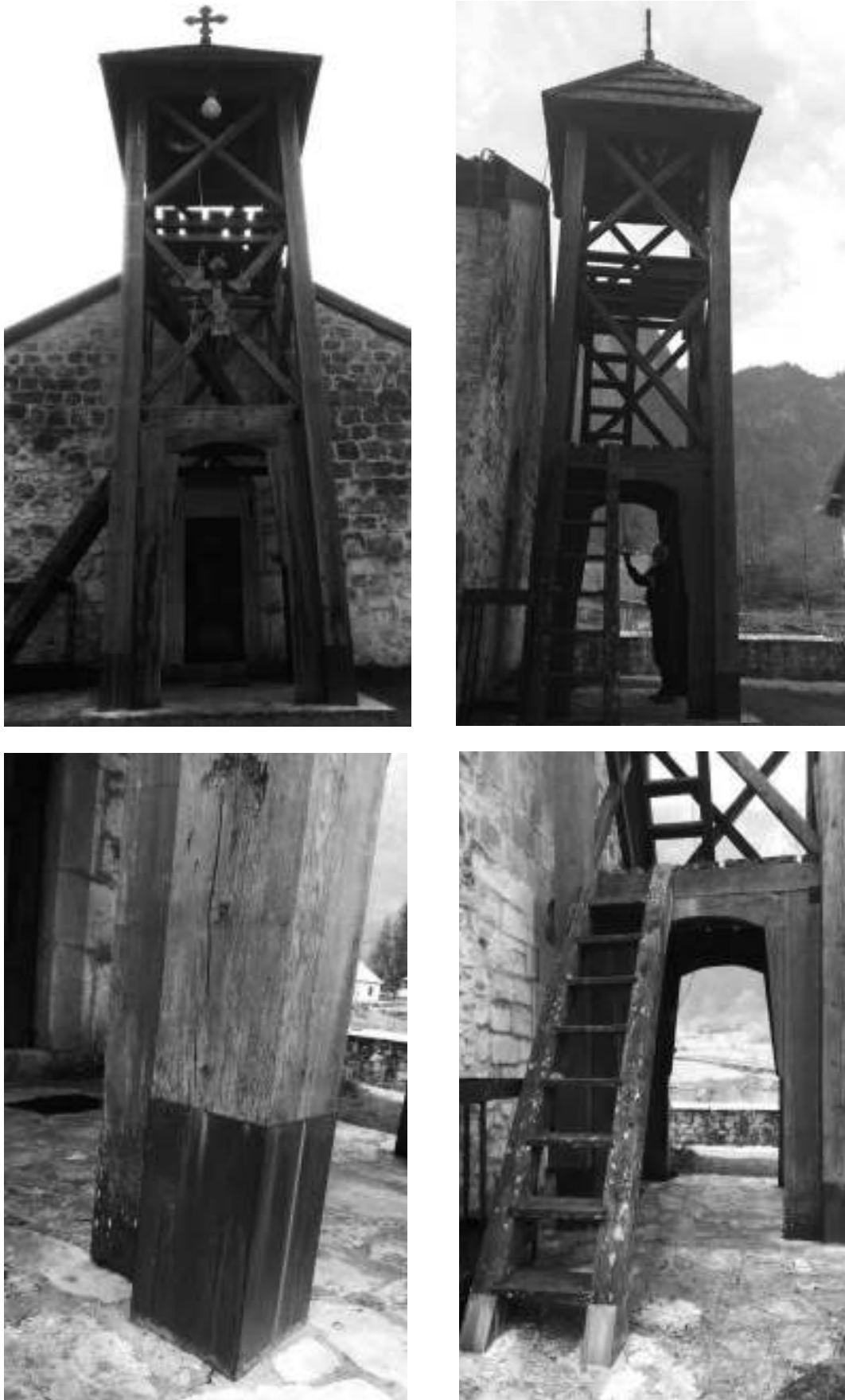
Figure 7: Wooden bell tower of Monastery Dobrilovina
