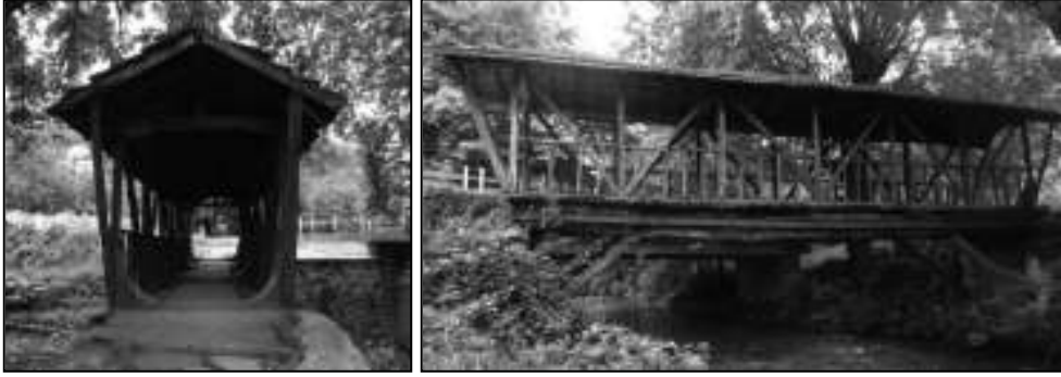
Figure 16, Figure 17: Historical Yakaören Bridge in Kastamonu (Photographs taken by S.Yılmaz, June 2016)
