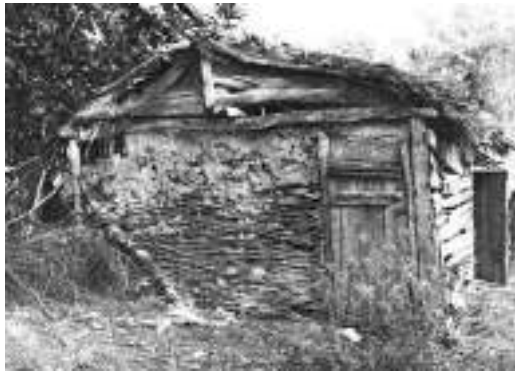
Figure 16: Interlaced twigs on a timber skeleton rural building (Yakar, J., Garson, J. L.) Figure 17: An example of an advanced Baghdadi lath system (Drawing: Dışkaya, H.)
