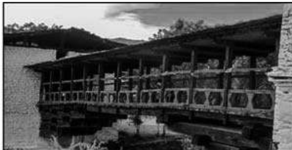
Figure 4: Cantilever Timber Bridge In Bhutanese [3].
