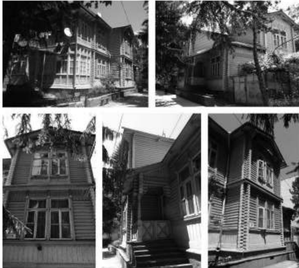
Figure 7: Log house. Rustaveli str. 117, Borjomi
