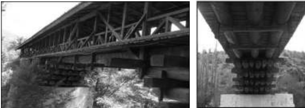
Figure 23,24: Historical Bayramören Bridge in Çankırı (After restoration)[16].
