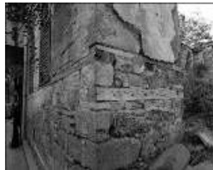
Figure 11: An 18 th Century wall detail in Antalya (Photo: Dışkaya, H.)
