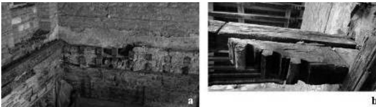
Figure 4. a. The remains of the original timber 1 st floor, trapped inside the southern wall. To the left, the in situ 1 st beam (with another beam placed over it, probably during the Ottoman period). b. The remains of the 12th beam, with its southern corbel and underlying cornice/tie beam
