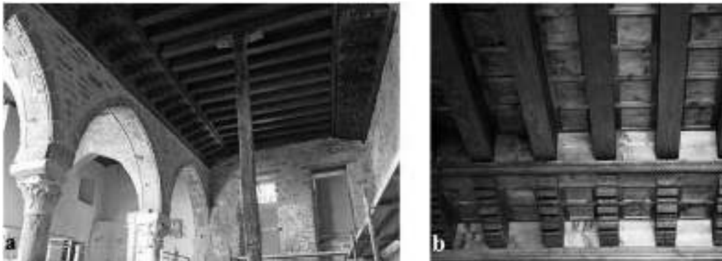
Figure 11. a. The reconstructed floor. The Ottoman era support column made of a reused Venetian beam was put back into place, as an important testimony of the building’s construction history. b. Closeup of ceiling
