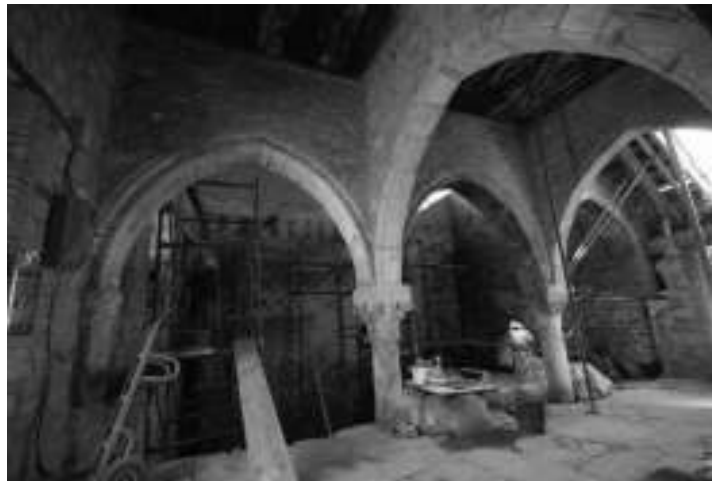
Figure 2. The gothic Venetian loggia looking from the north, during restoration work. The two transversal arches are Ottoman era additions. The transversal Ottoman-era wall within the loggia has already been removed
