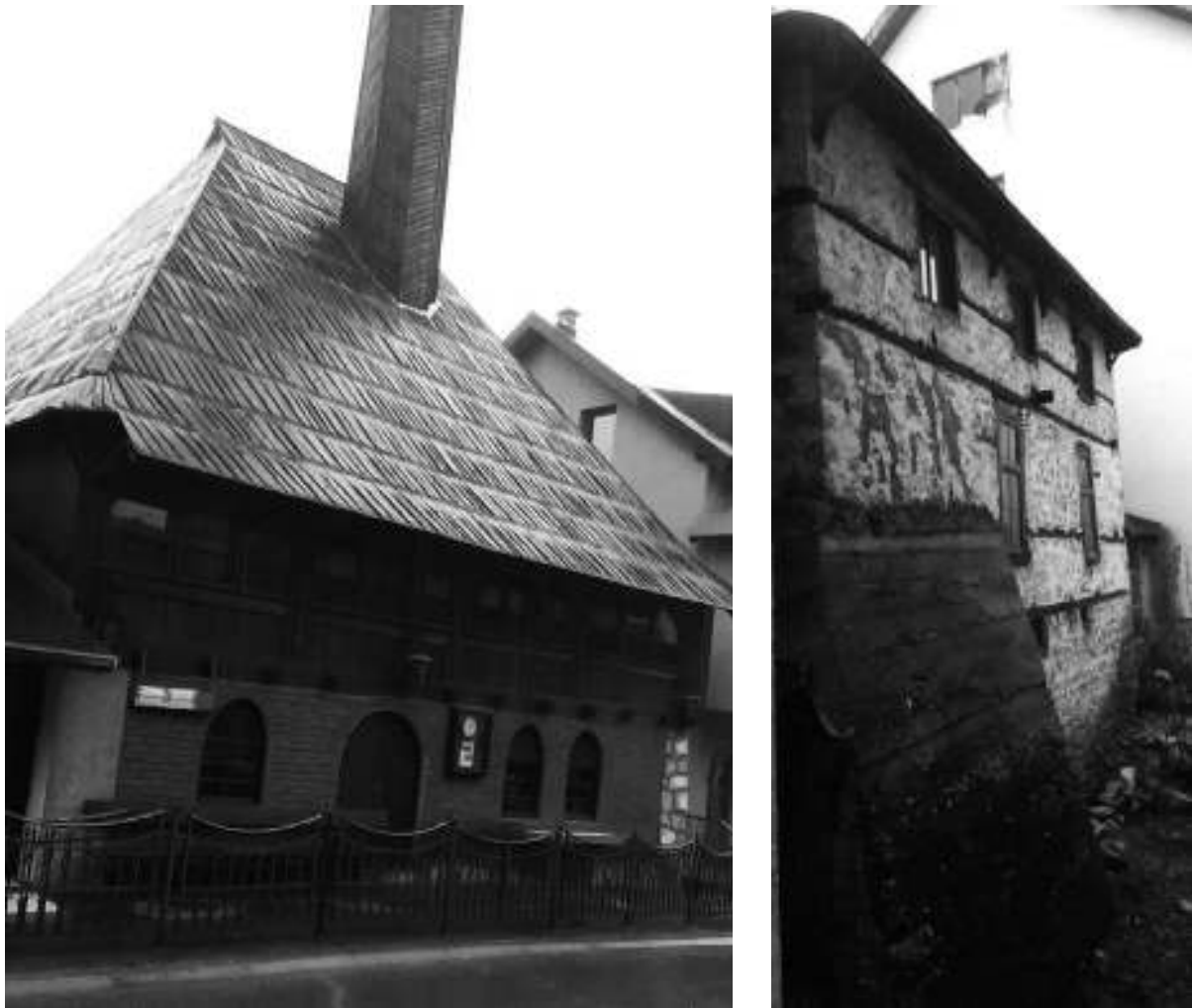
Figure 4: Details of frontal and rear façade of Kučanska Mosque – current state
