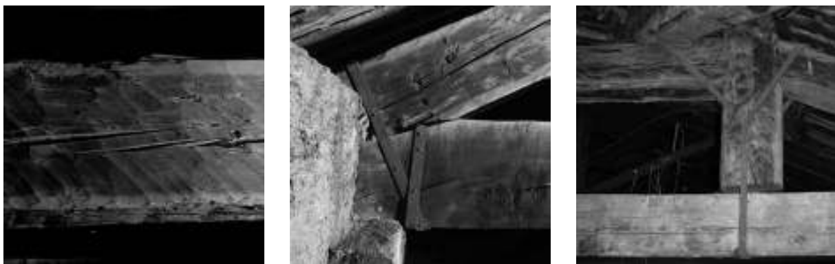
Figure 5: On the left: traces of hand working with the hatchet that can be seen with raking light.
