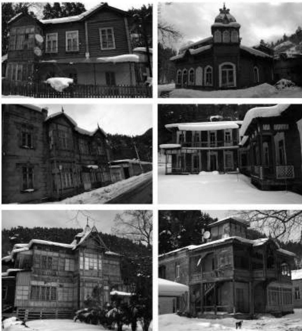
Figure 10: Abastumani. Heritage Buildings with timber structures
