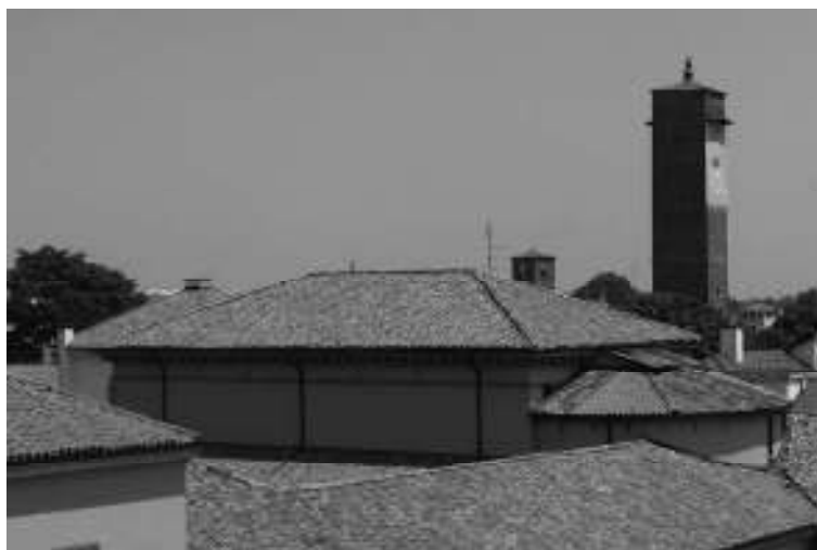
Figure 2: The Great Hall photographed from south-west. We can see the hipped roof of the hall and the roof of the apse shaped as a truncated cone with a single pitch covering the former skylight (photo by E. Zamperini).
