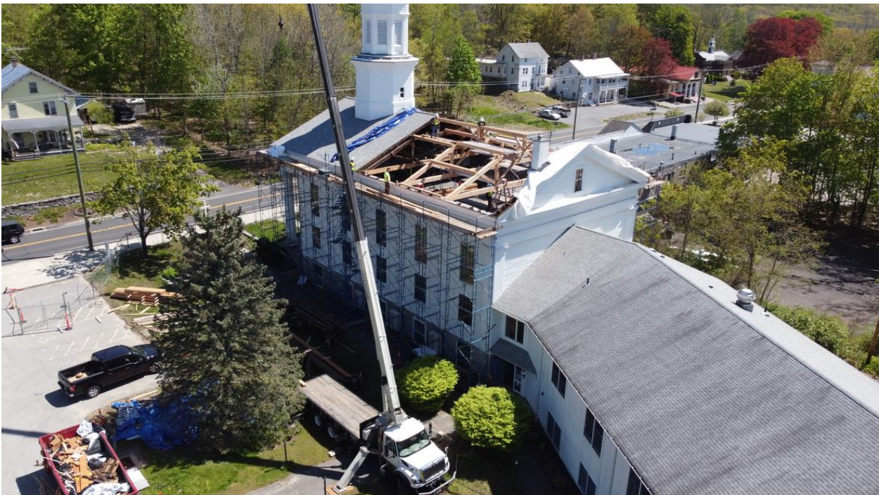
Figure 2: Repair Work Underway – following methodology determined by IPM.
