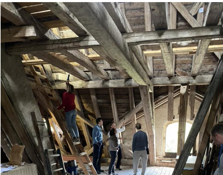
Figure 1: Timber roof structures of Louhisaari Castle. Photo: Panu Savolainen.
