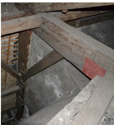
(a) View on site
