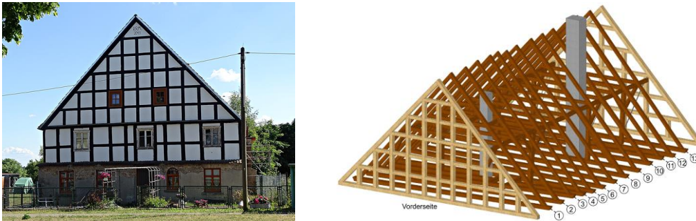
Figure 1: Exterior view of the aisled house (left) and isometric view on the roof construction (right)
