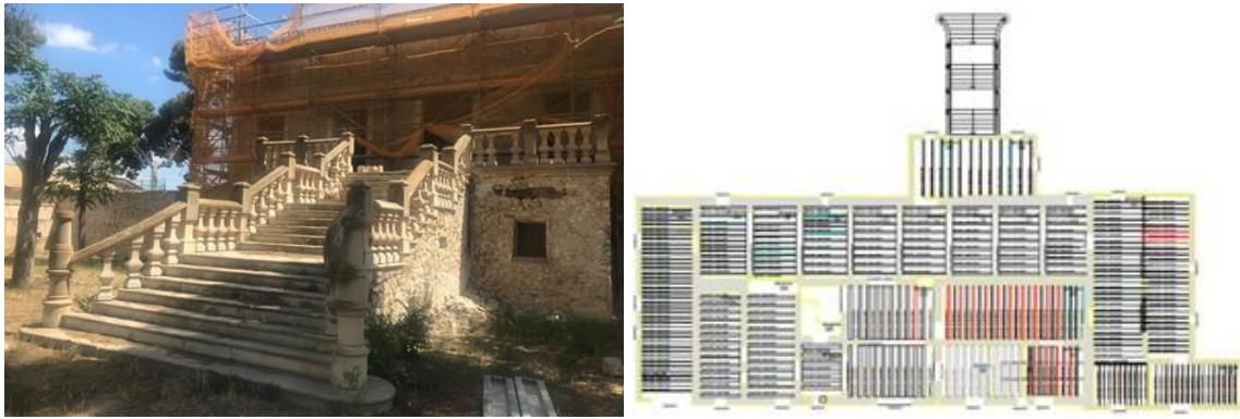
Figure 1: North façade (left) and ground floor (right) of the building
