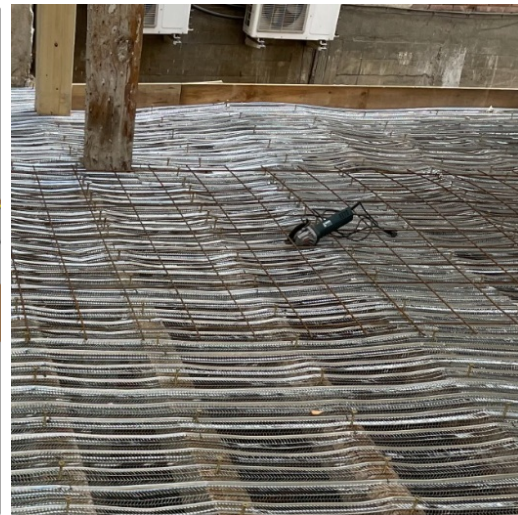
Figure 4: Laying of the mixed floor slab.
