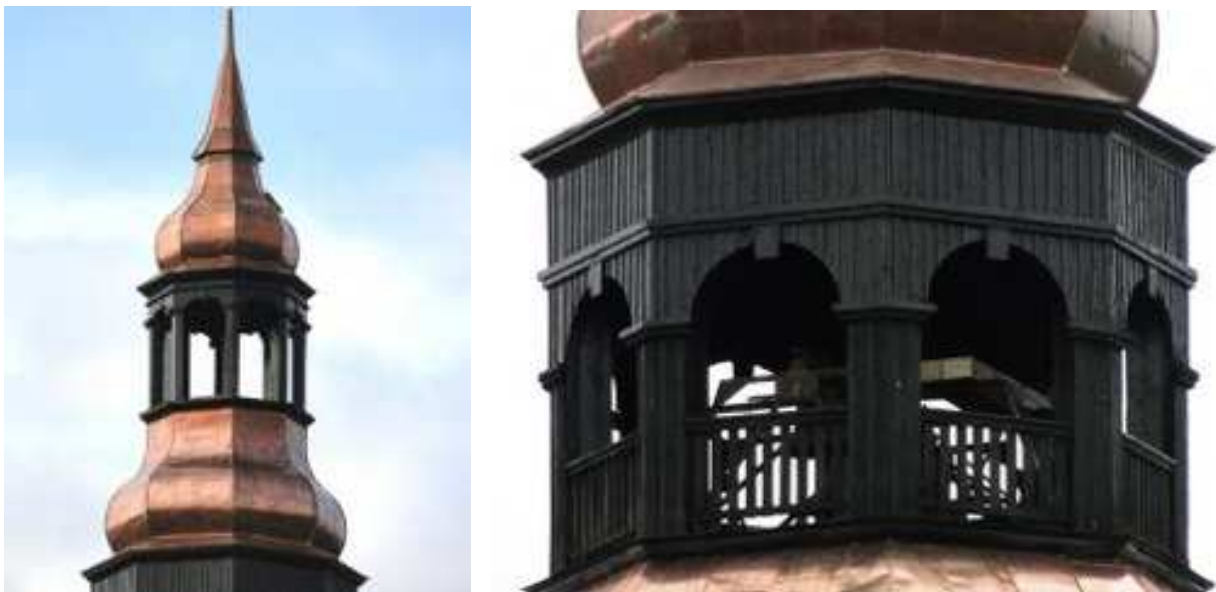
Figure 5: Upper (left) and lower (right) lantern of the tower after works
