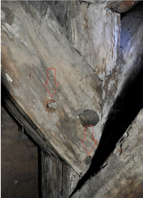
Fig. 4. Toruń, 6 Mostowa Street. Roof structure of building C. Traces of raft floating of the building material (Photo by U. Schaaf).
