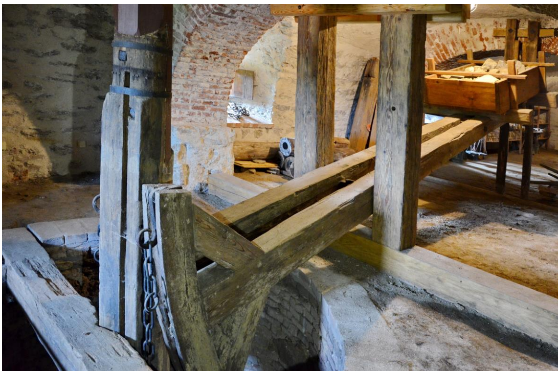
Figure 4: Lifting mechanism in lowered position. Hinge of the principal post in foreground, counterweight box in the background, photo Jiří Bláha, 2022.
